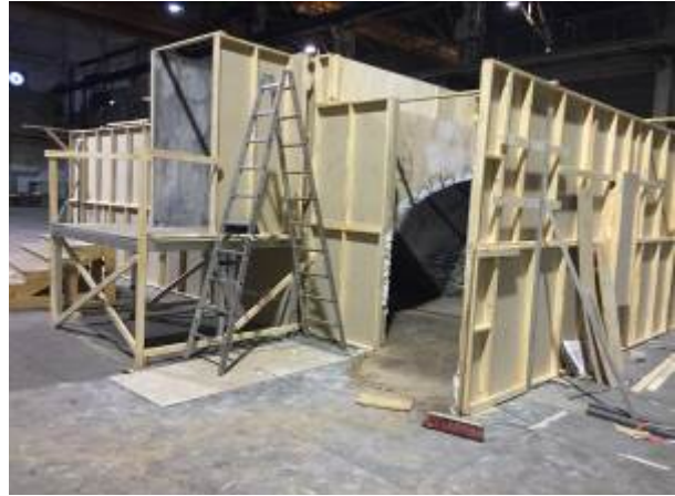
Studiobau in der Marlene Dietrich Halle in Potsdam
